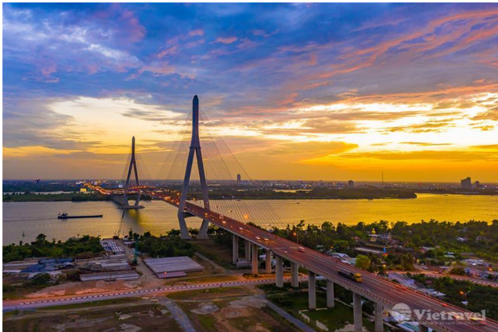
Figure 4.4 Can Tho Bridge
